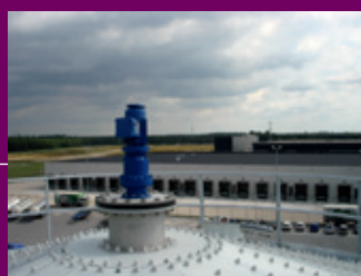
AFR reactor at ITC Holland Transport bv, with a capacity of 4200 kg COD/d
