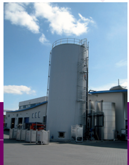
AFR reactor at ITC Holland Transport bv, with a capacity of 4200 kg COD/d
